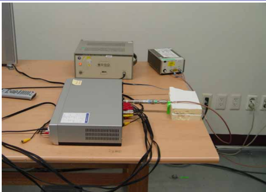
Picture 7. Ant. Transfer Switch
