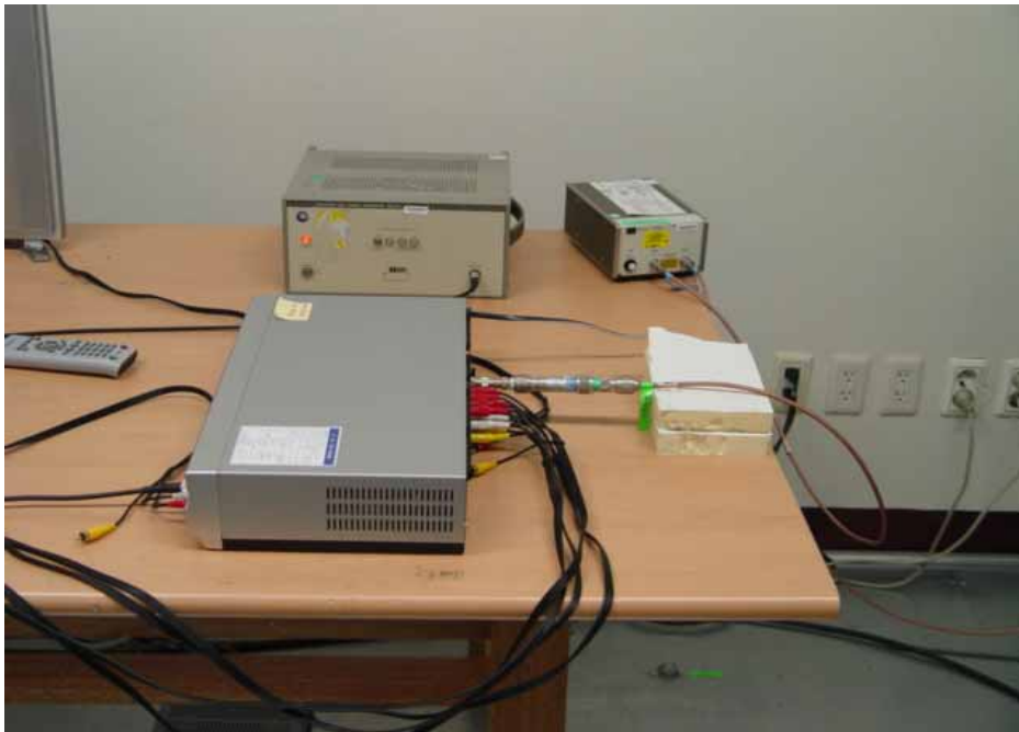
Picture 7. Ant. Transfer Switch
