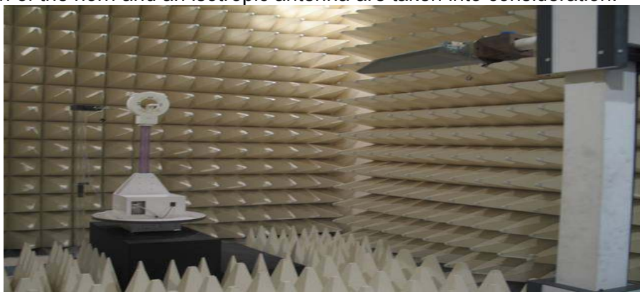
Figure2. Photograph of 3m Fully-Anechoic Chamber
