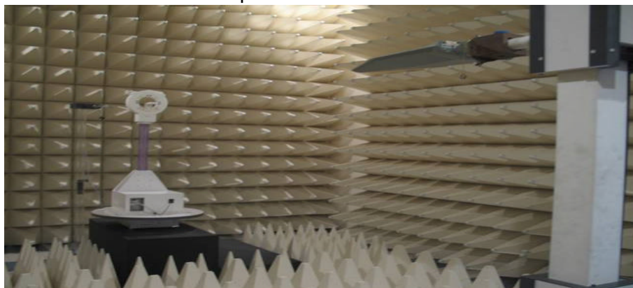
Figure2. Photograph of 3m Fully-Anechoic Chamber
