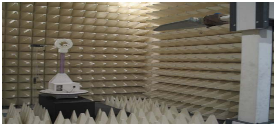
Figure2. Photograph of 3m Fully-Anechoic Chamber
