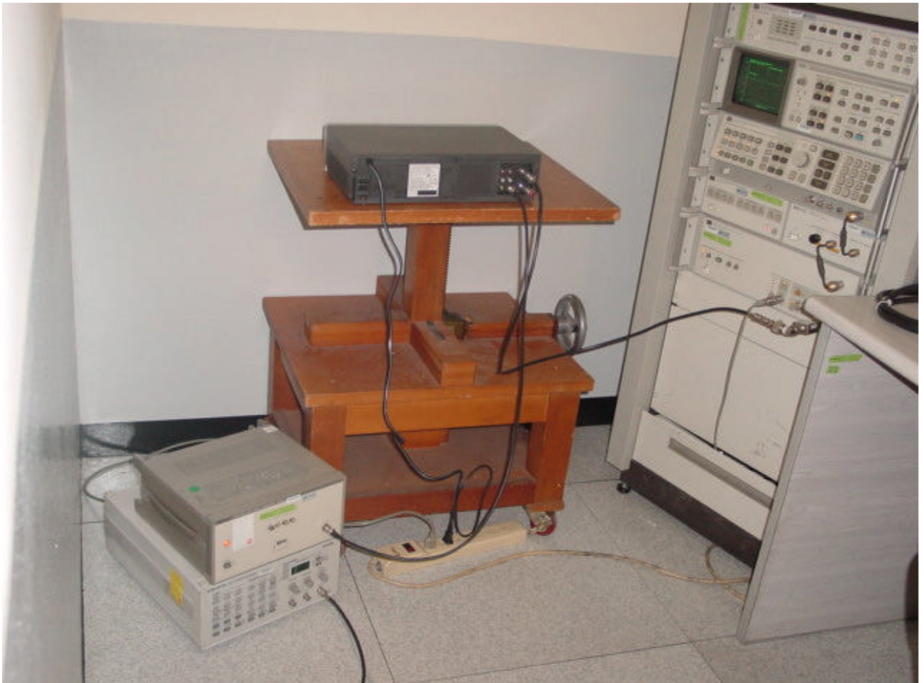
Fig. 4 Test Setup for Antenna Transfer Switch Measurement
