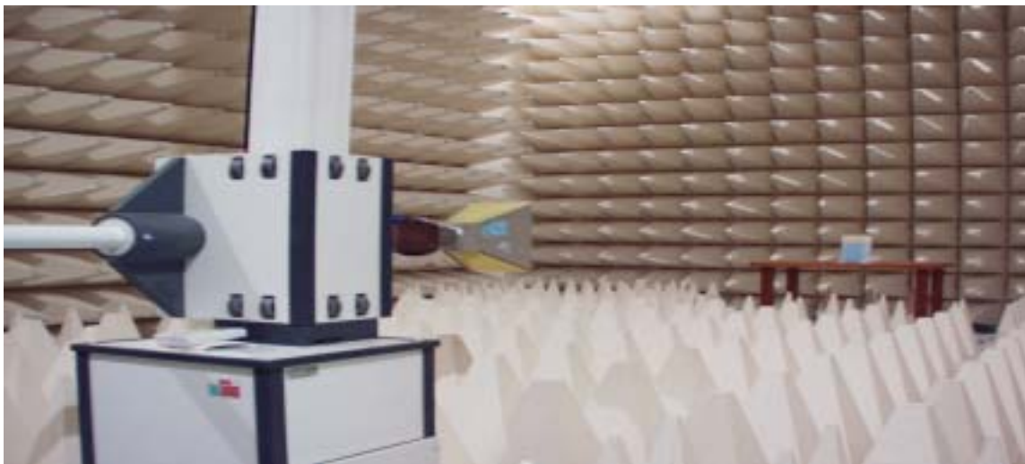
Figure2. Photograph of 3m Fully Anechoic Chamber
