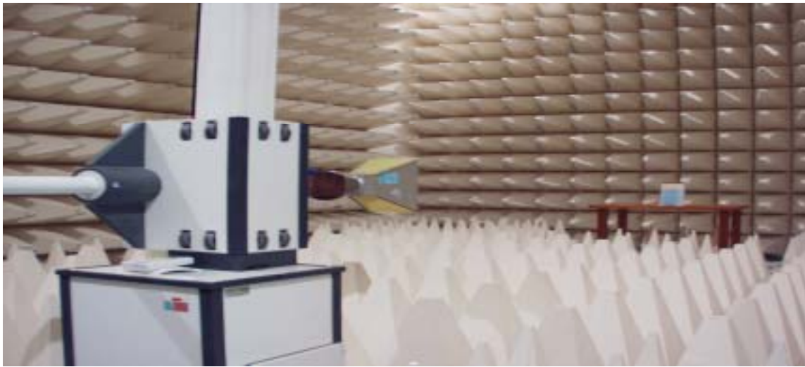
Figure2. Photograph of 3m Fully Anechoic Chamber
