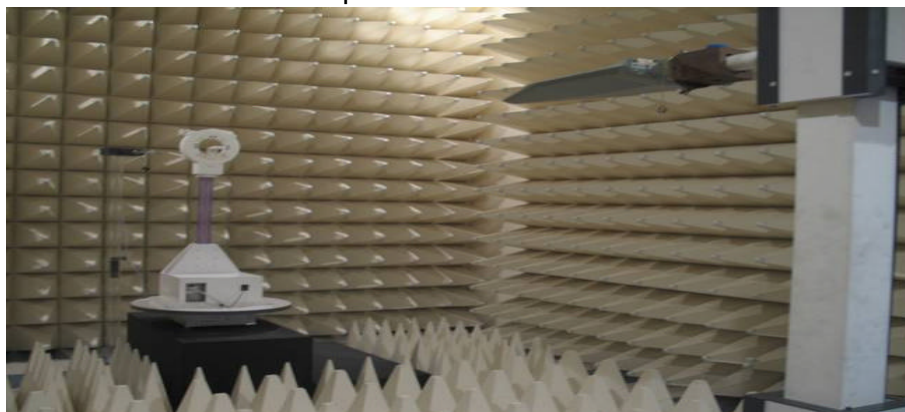
Figure2. Photograph of 3m Fully-Anechoic Chamber
